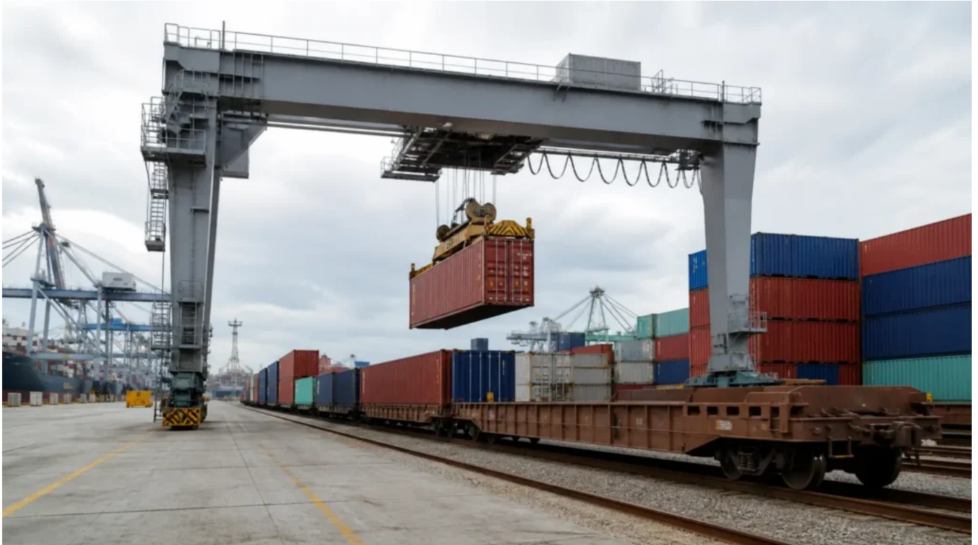
Handling on the SGN air / Cat Lai sea routing serving Ho Chi Minh City.
