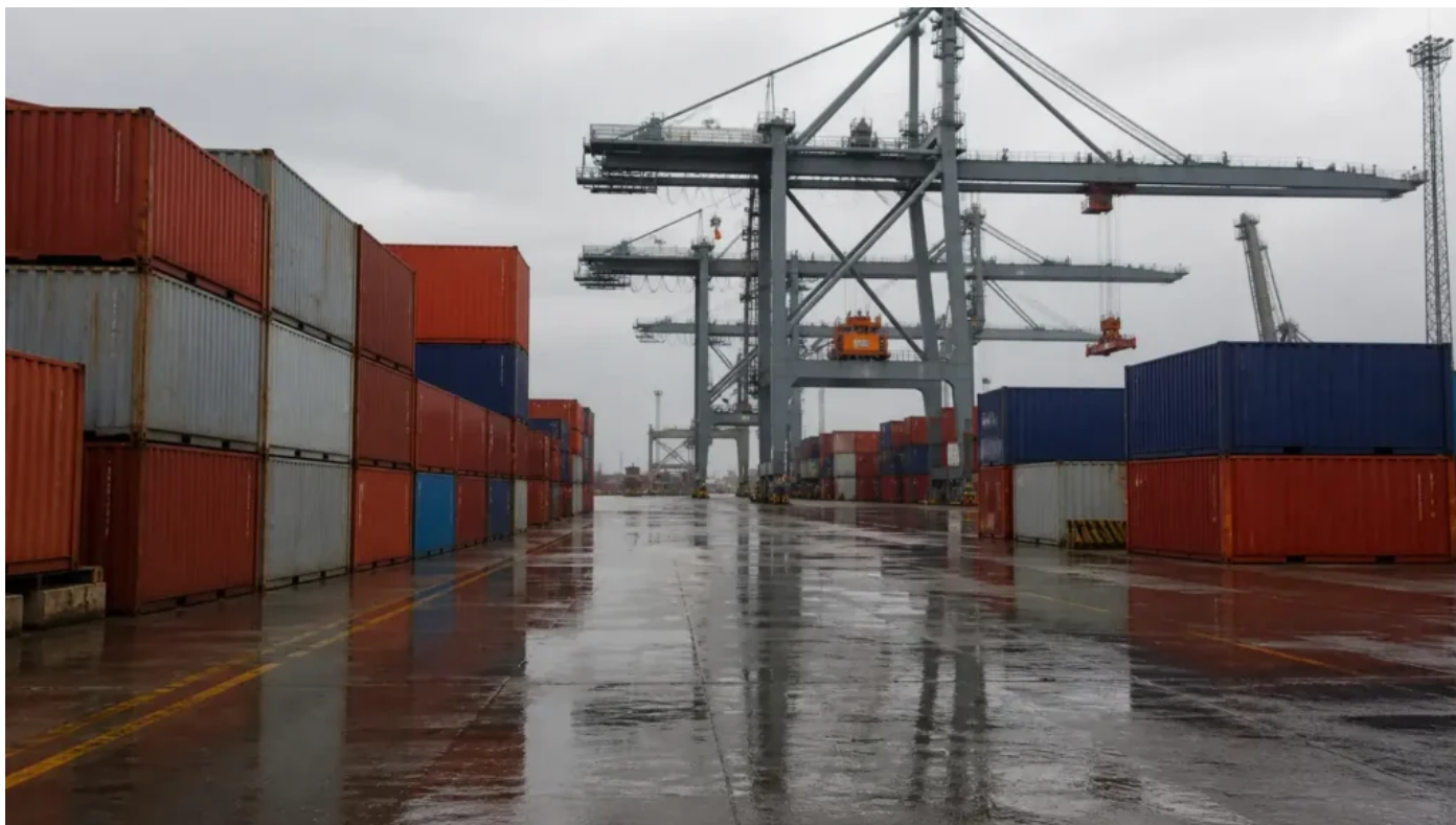
Cargo handling on the China-Kocaeli lane.
