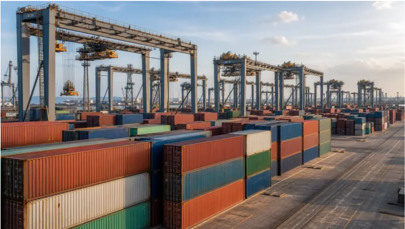
Handling on the HIR air / Honiara sea routing serving Honiara.
