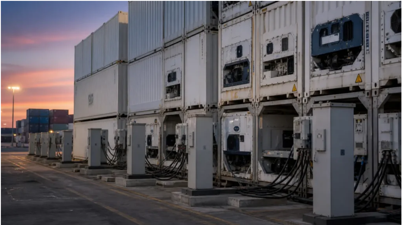
Handling on the LIM air / Chancay sea routing serving Chancay.
