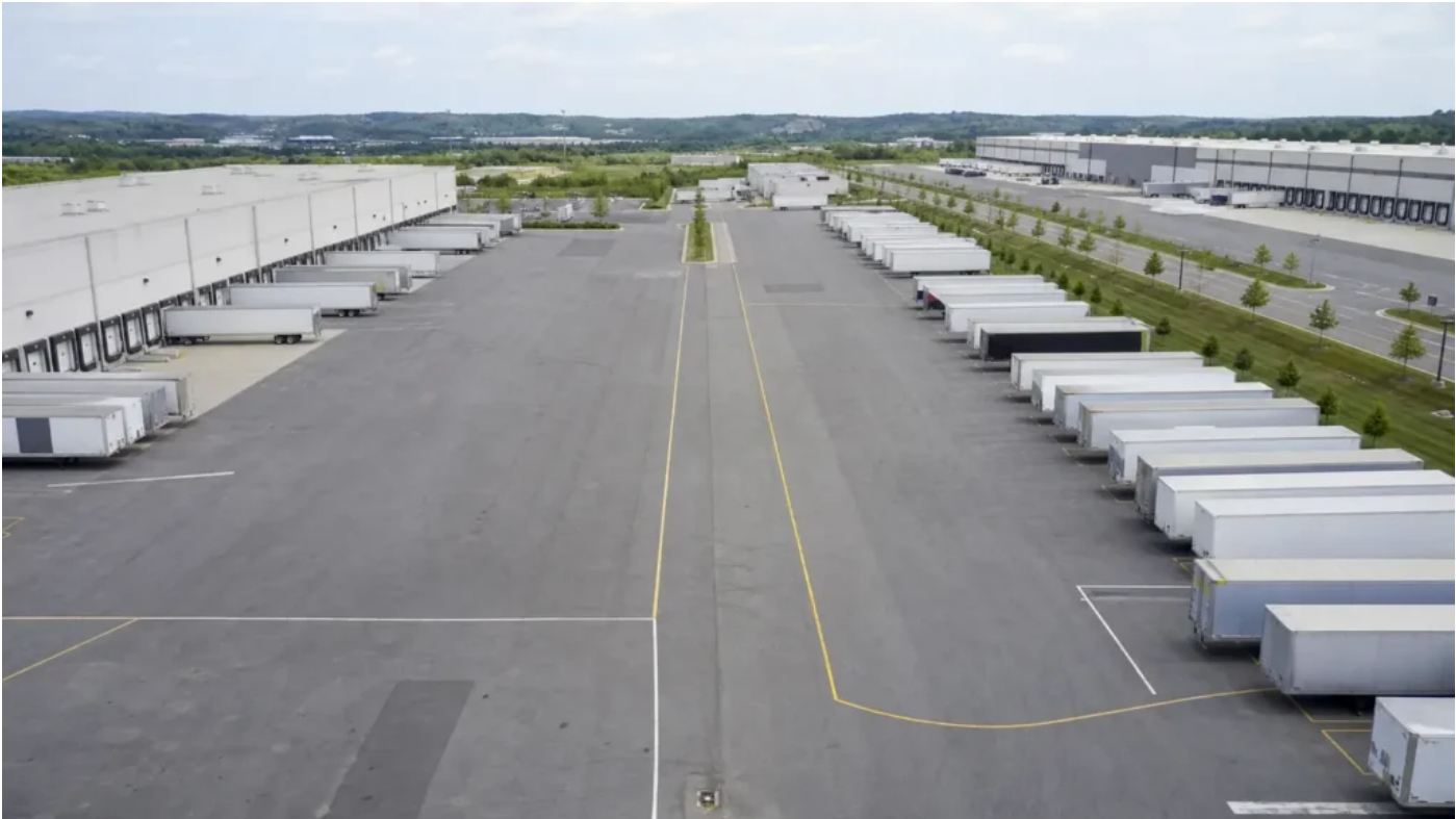
Handling on the TIV air / Bar sea routing serving Herceg Novi.
