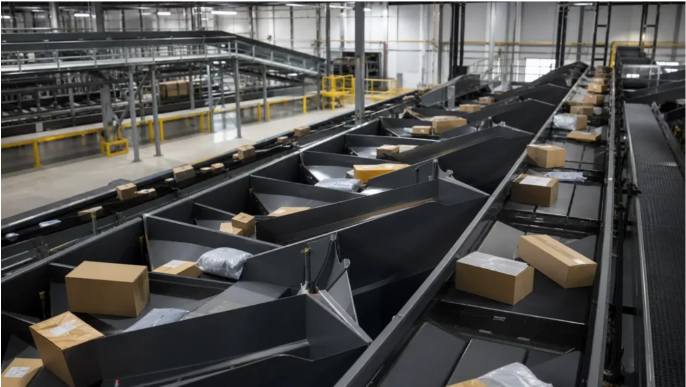
Handling on the PUJ air / Caucedo sea routing serving Punta Cana.
