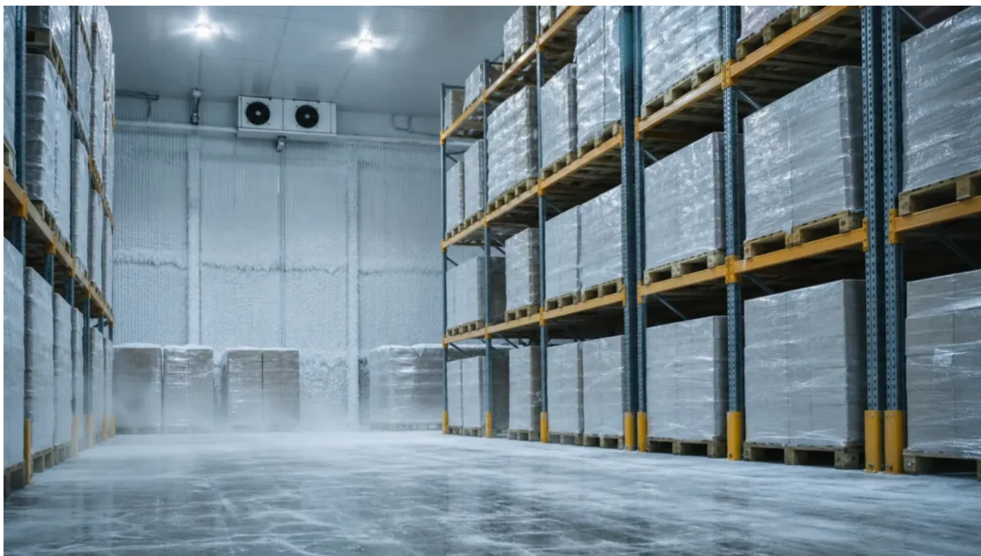
Handling on the EVN air / Poti transit routing serving Vanadzor.
